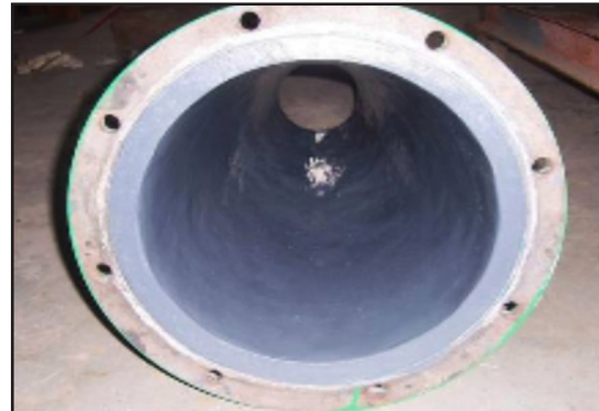
Repaired exit cone
